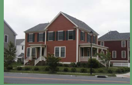
Attached single-family, like this duplex above, can resemble a single-family home.
