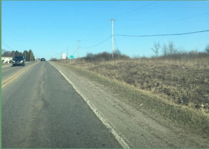
Roadside stormwater drains reduce the effects of heavy rainfalls and flooding throughout the Township, and should be protected from encroaching agricultural activities.
